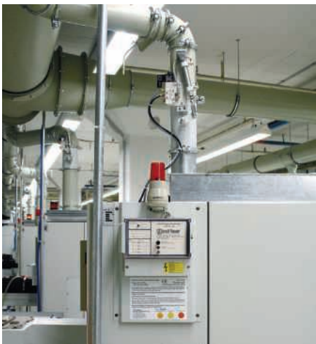
Control system for automatic fire system in conjunction with mist extraction protection
