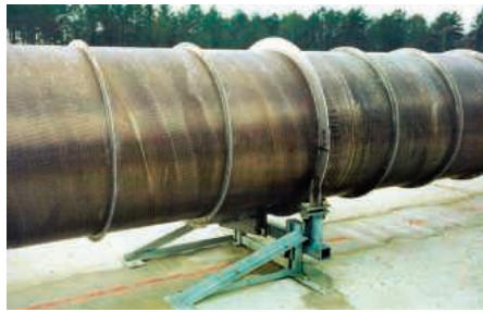
A LIGO spiral-welded beam tube after assembly at Livingston (Photo courtesy of: Caltech/MIT/LIGO Lab)
